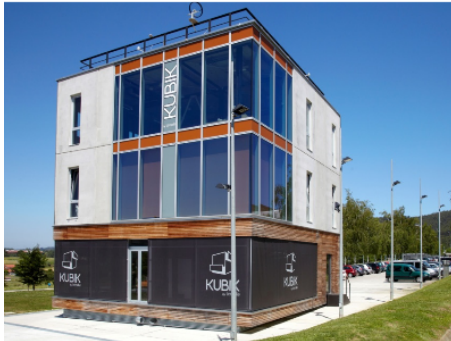
Figure 6: KUBIK Smart Building
